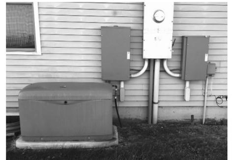
power goes out. They run on propane or natural gas and cost \$3,000 to \$6,000, not including installation. Do not try to install a standby generator on your own; they should be installed by an experienced electrician.
